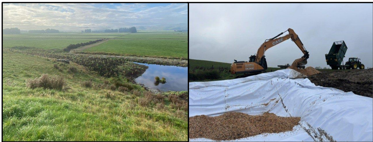
Figure 2 – Wetland Enhancement and Construction of the Woodchip Biofilter
